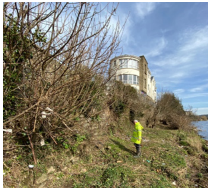
Wall where vegetation clearance was undertaken
