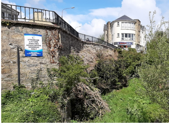
Wall on left bank downstream of Lifford Bridge
